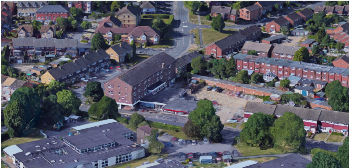
Figure 1 Aerial view of Dale Court and No150 and No146-148 Haines Way
